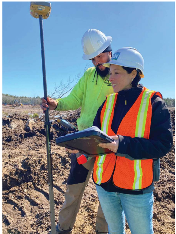
Sara daSilva Quintal, BBC's Restoration Ecologist, discusses earth moving and wetland re-creation with Mattapoisett Bogs restoration contractors at Luciano's Excavating of Taunton.
