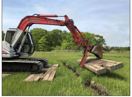
Bucket teeth used to create new / clean out existing runnels
